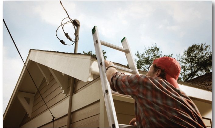
Ladders placed too close to power lines become dangerous conduits of electricity. Source: Touchstone Energy® Cooperatives
