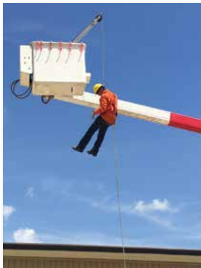
OEC lineman Ben Wilcox practices rescuing himself from the truck bucket.
