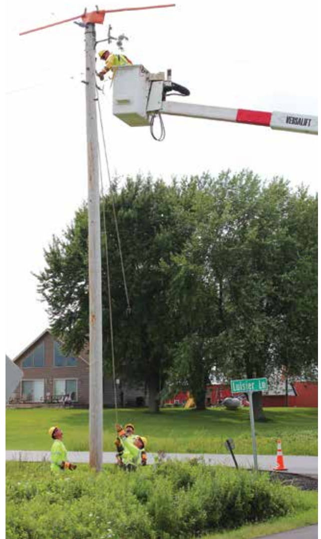
An OEC crew works to fix power lines that were recently taken down by an airplane that was dusting farm fields.
