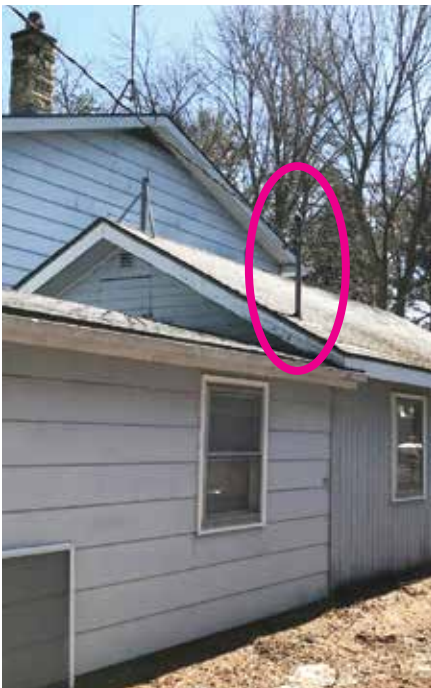
Photo on the left: The service going into the home is circled. Can you see the meter? No. The meter is inside of the property and not properly installed where it is accessible. Middle: The path to the meter is blocked. Photo on the right: We can’t safely get into the meter that is surrounded by decking.
