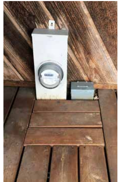
Photo on the left: The service going into the home is circled. Can you see the meter? No. The meter is inside of the property and not properly installed where it is accessible. Middle: The path to the meter is blocked. Photo on the right: We can’t safely get into the meter that is surrounded by decking.
