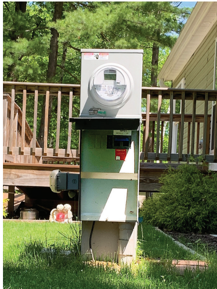
When you call in an outage, you will be asked if you checked your main breaker. Be aware that some types of service hook-ups have a main breaker underneath or next to the meter.
