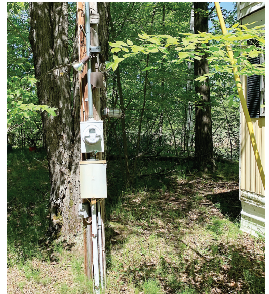
When you call in an outage, you will be asked if you checked your main breaker. Be aware that some types of service hook-ups have a main breaker underneath or next to the meter.
