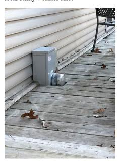
Meters should be located so accessibility will not be obstructed by future alterations or additions.
